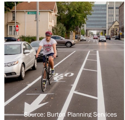
Example of a buffered on-street bike lane
