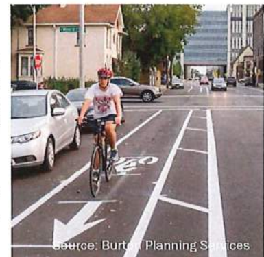
Example of a buffered on-street bike lane
