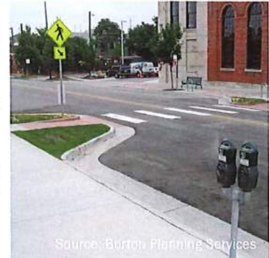
Example of a sidewalk bulb-out
