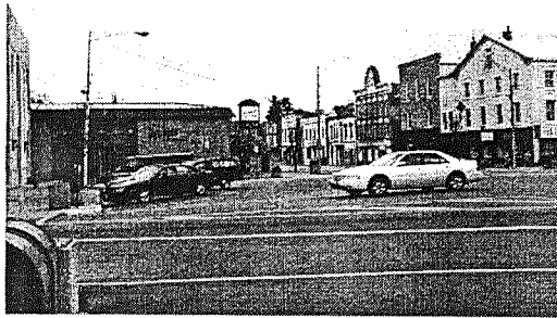
Incompatible New Building Addition - Scale, Character and Materials
