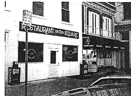
Incompatible Change to the Original Storefront
