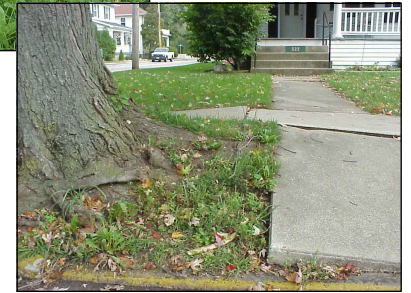
BLOCKS, OR PORTION OF BLOCKS, THAT CAUSE AN ABRUPT CHANGE OF 1 INCH PER FOOT (OR MORE) IN ANY DIRECTION OF THE SIDEWALK.
