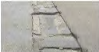
EXAMPLE: Large Holes in Surface
