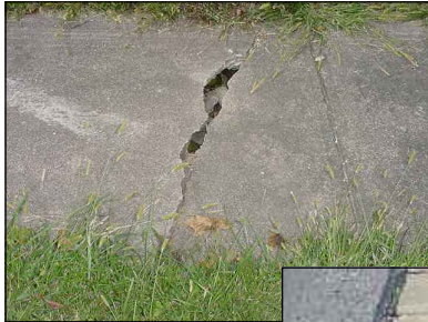
ANY SIDEWALK BLOCK (BASED ON 20 SQ. FT.) HAVING A CRACK OR CRACKS IN IT OF AT LEAST 1/2 INCH WIDE WITH A MINIMUM OF 4 LINEAL FEET IN ONE BLOCK. (VARIOUS SIZE BLOCKS WILL BE EVALUATED PROPORTIONALLY.)
