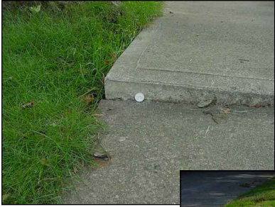
ADJOINING BLOCKS OR PORTIONS THEREOF WHOSE EDGES DIFFER VERTICALLY BY MORE THAN 1/2 INCH.
