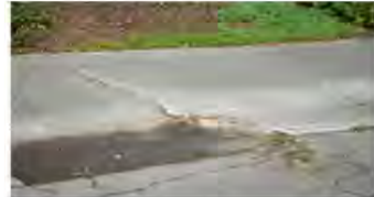
EXAMPLE: Asphalt repairs
