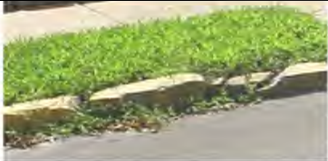
EXAMPLE: Settlement / Vertical Offset
