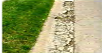
EXAMPLE: Exposed aggregate
