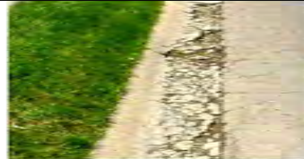
EXAMPLE: Exposed aggregate
